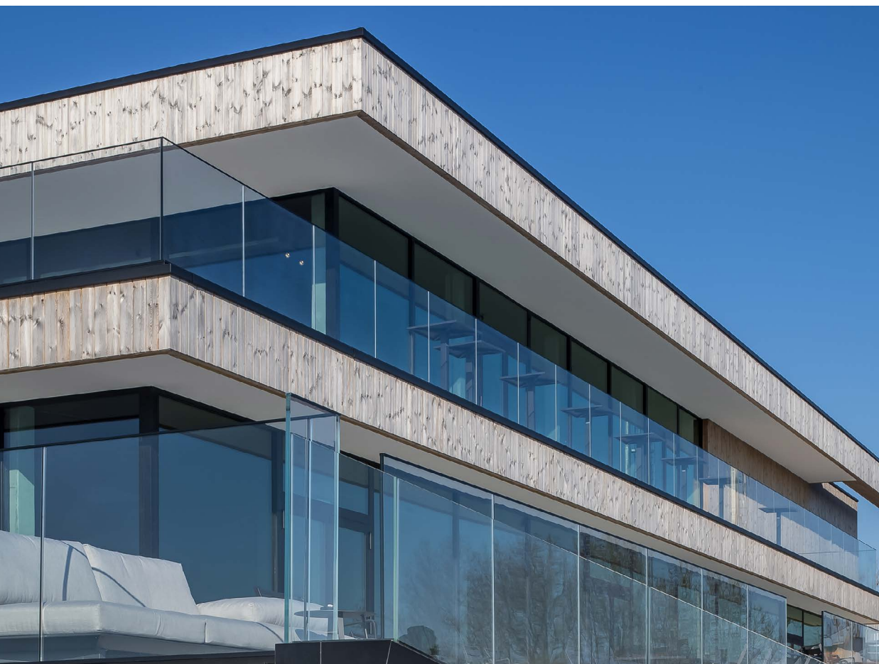
Project Hockey & Padel Gantoise, Gent. Gevelbekleding in LDCwood® ThermoWood® grenen, brandvertragend behandeld door Lemahieu Fire Protection® with Burnblock® tot B-s1,d0.
