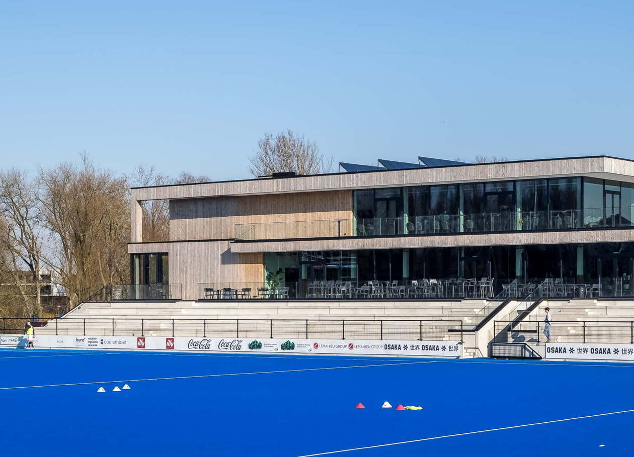
Project Hockey & Padel Cantaise, Gent. Gevelbekleding in LDCwood® ThermoWood® grenen van LDCwood, brandvertragend behandeld door Lemahieu Fire Protection® with Burnblock® tot B-s1,d0.
