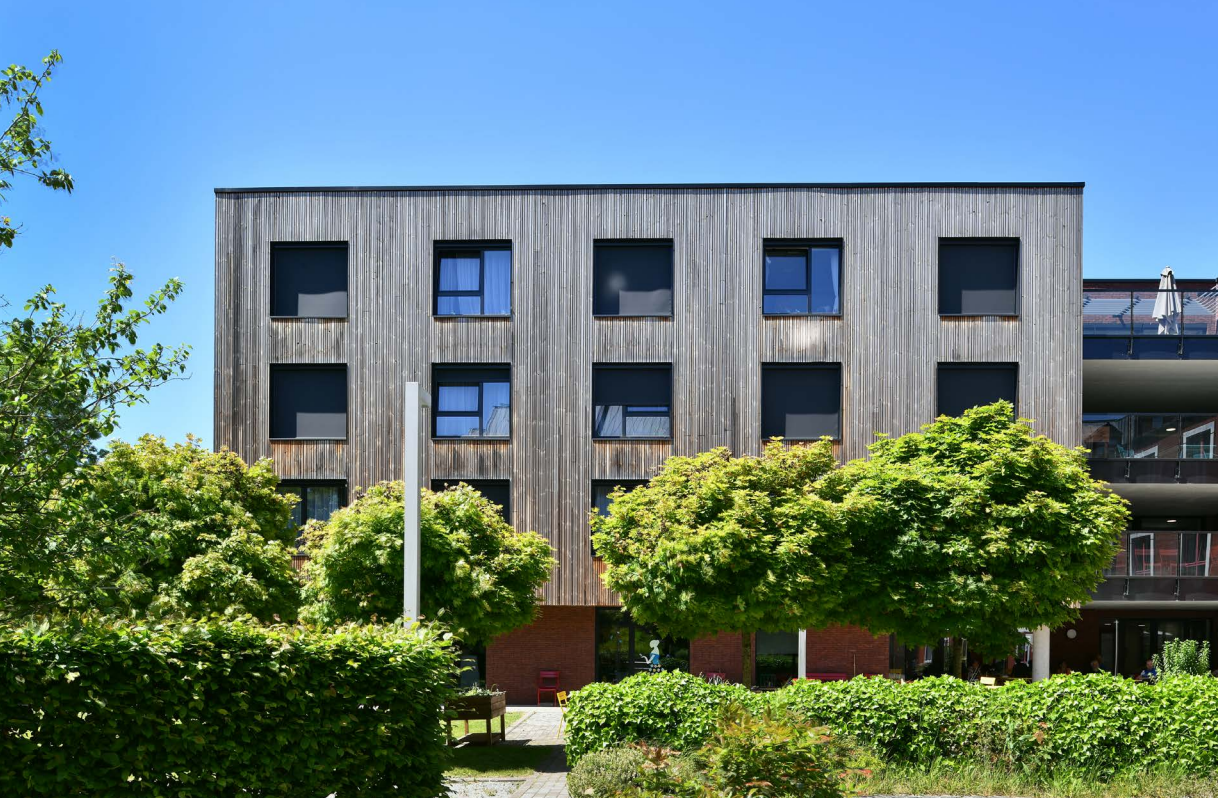
Project: Nursing home, Couillet. Facade cladding in planed LDCwood® ThermoWood® Pine treated with fire retardant by Lemahieu Fire Protection® with Burnblock® up to the requested reaction to fire class.
