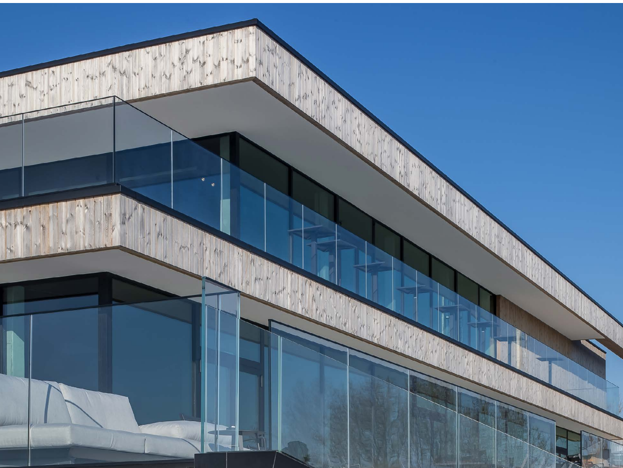
Project Hockey & Padel Gantoise, Ghent. Facade cladding in LDCwood® ThermoWood® Pine, treated with fire retardant by Lemahieu Fire Protection® with Burnblock® up to B-s1,d0.
