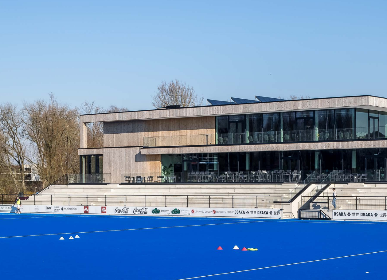
Project Hockey & Padel Gantoise, Ghent. Facade cladding in ThermoWood® pine by LDCwood, treated with fire retardant by Lemahieu Fire Protection® with Burnblock® up to B-s1,d0.
