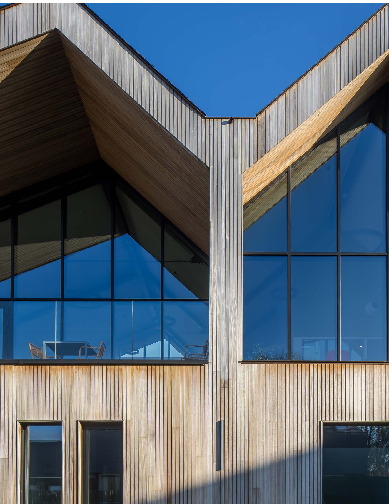
Project: WZC Wielkine, Nazareth. Facade cladding in ThermoWood®, treated with fire retardant by Lemahieu Fire Protection® with Burnblock® up to B-s2,d0.
