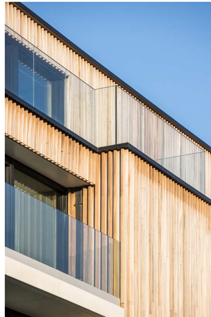
Project: residentie Oasis Wenduine, gevelbekleding in LDCwood® ThermoWood® ayous.
