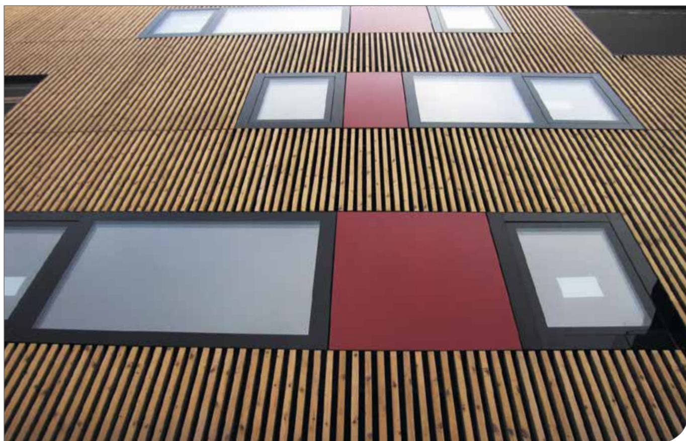
Figure 62. Exterior cladding made of ThermoWood® products.
