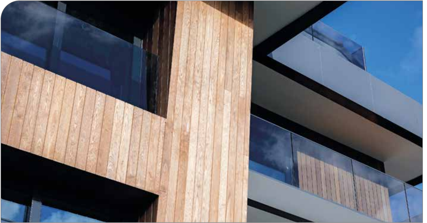
Figure 60. Exterior cladding made of ThermoWood® products. (Turkey).
