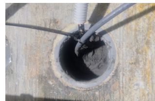
Application SEAL-ALL® AQUABLOCK
